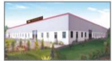
Manufacturing Unit-VI, Nalagarh (Himachal Pradesh)
