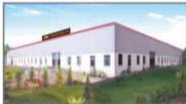
Manufacturing Unit-VI, Nalagarh (Himachal Pradesh)
