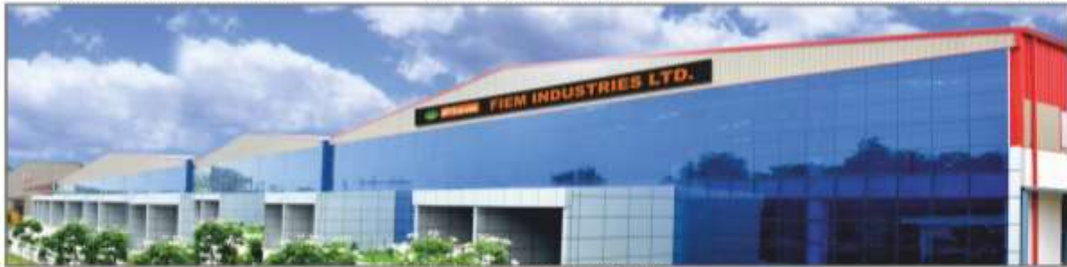
Manufacturing Unit-VIII, Tapukara (Rajasthan)
